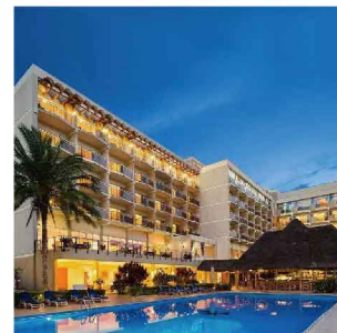
Kitchen Exhaust Purification Project, Rwanda
