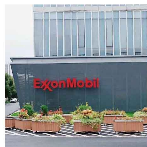
ExxonMobil Office, Shanghai, China
