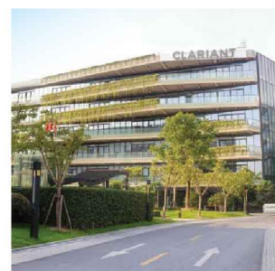
Clariant Chemicals Office, Shanghai, China
